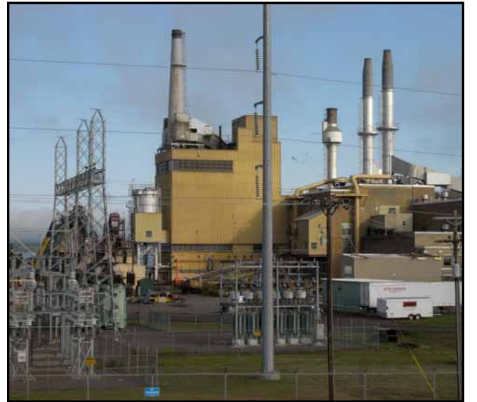
The power plant in Ashland, Wisconsin has an output capacity of 76 megawatts. 11
