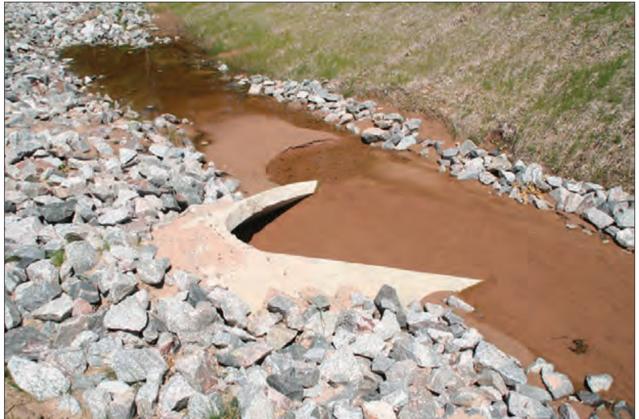
Undersized sedimentation basin along a mine haul road. The sediment will need to be removed for the basin to work as intended.
